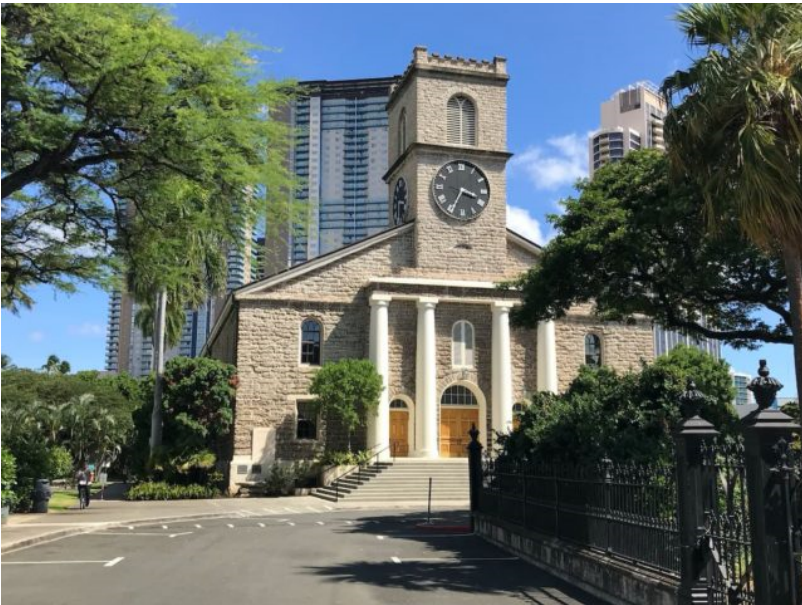
The oldest church in Honolulu, the Kawaiahaʻo Church, on Oʻahu Island, built 1836–1842 from coral reefs
